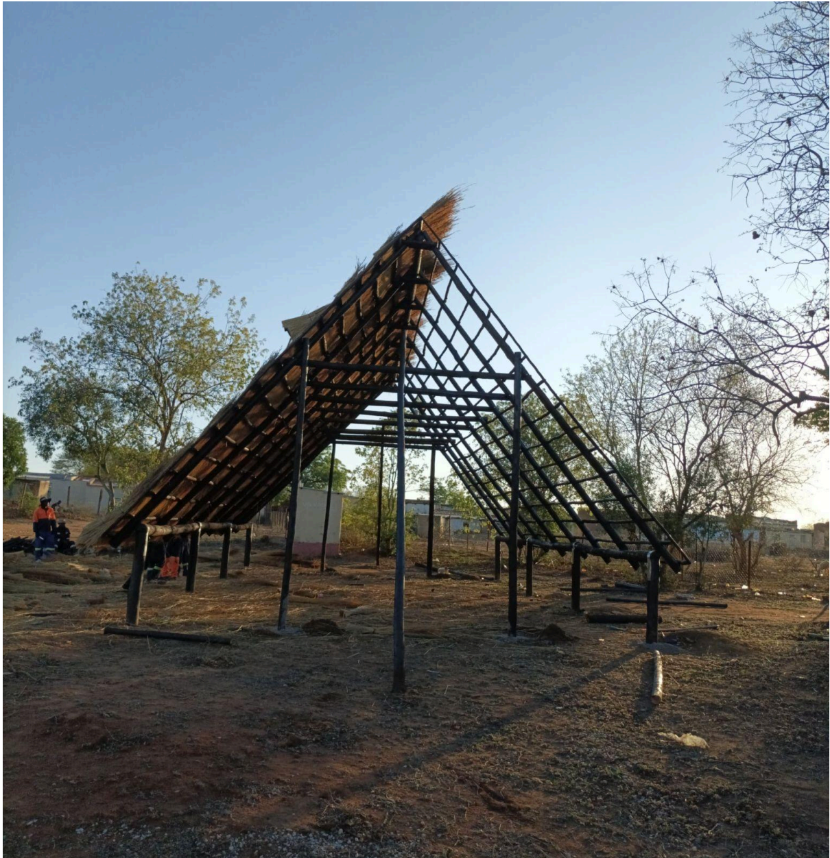
Second roof thatching
